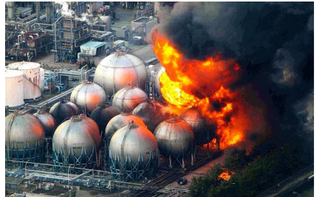
Cosmo Refinery, Chiba, Japan – 2011 Tohoku Earthquake
